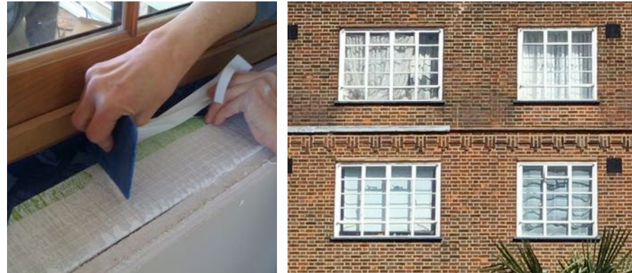
Replacement of windows is a key fabric efficiency measure. Single glazing should be replaced with double or triple glazing in every home. Measures to improve air tightness and reduce draughts require attention to the details when fabric works are undertaken.
