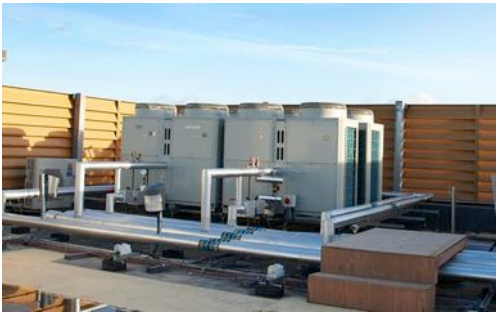
Left: A centralised heat pump system on the roof of a building. Right: Direct electric heating can use wall mounted radiators, panels or underfloor heating
